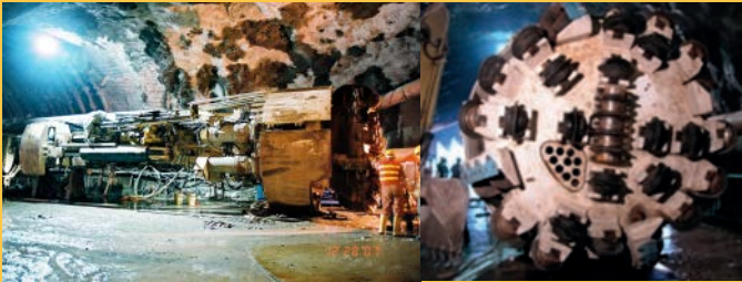
施工期間相片 Photograph taken during construction
